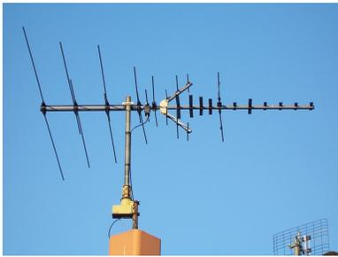
Unless you want to point your antenna in one direction and never move it, a rotor is a good investment. Seen to the left is a rotor attached to a pipe on the chimney. This allows the viewer in Bluffton to point the antenna toward us, towards Fort Wayne, or towards Toledo. A rotor costs about \$75 for a good quality device. Be sure to allow for a loop of Coax Cable when you go past the rotor, so the cable will not bind up and cause the cable to break.
